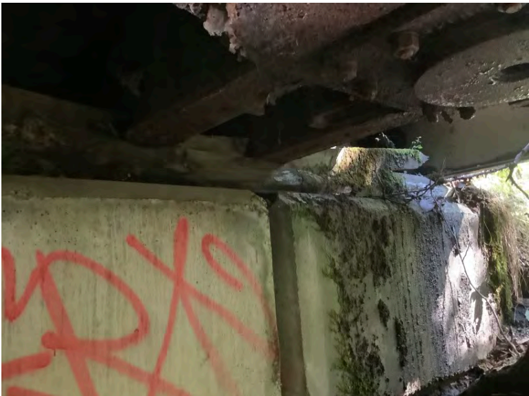
Left Bank Abutment when facing downstream
