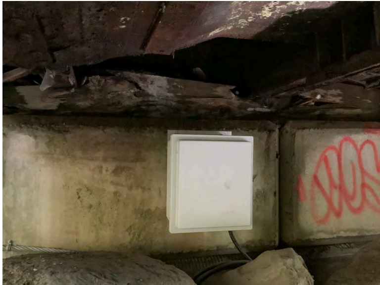
Left Bank Abutment when facing downstream
