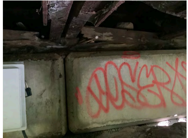
Left Bank Abutment when facing downstream
