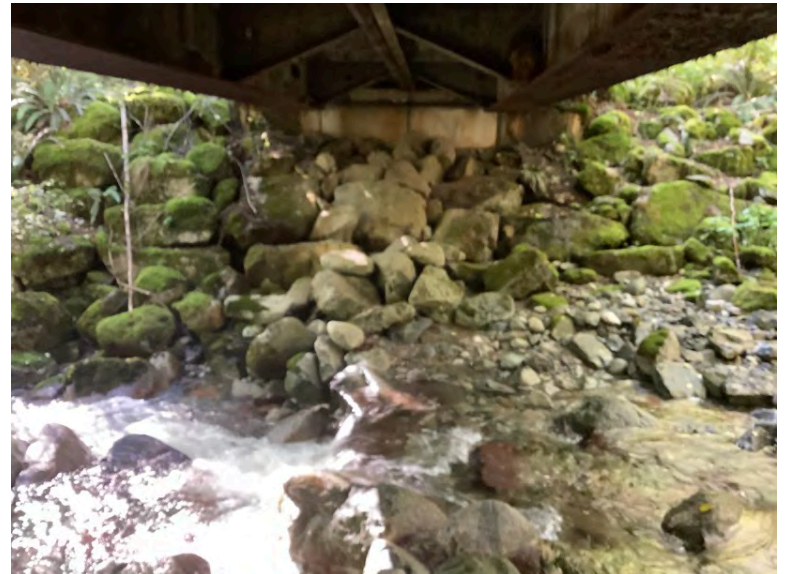
Right Bank Abutment when facing downstream
