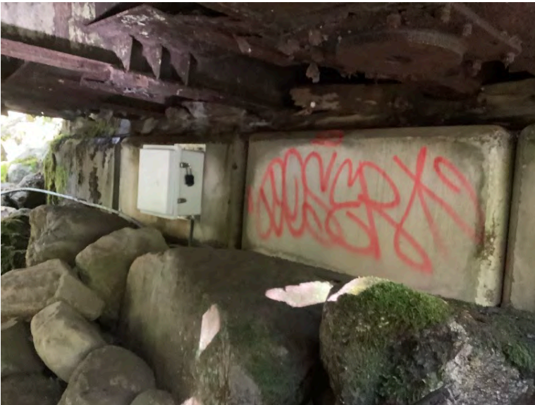
Left Bank Abutment when facing downstream
