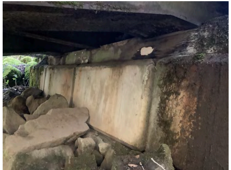
Right Bank Abutment when facing downstream
