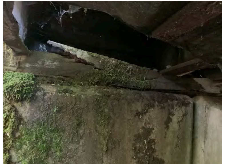
Left Bank Abutment when facing downstream
